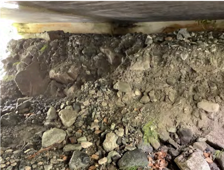
Right Bank Abutment when facing downstream
