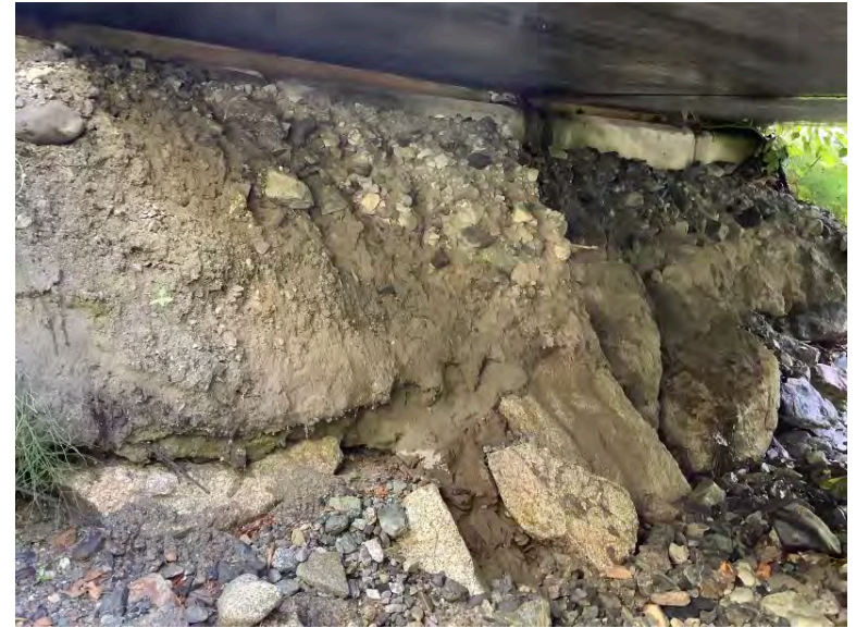
Left Bank Abutment when facing downstream
